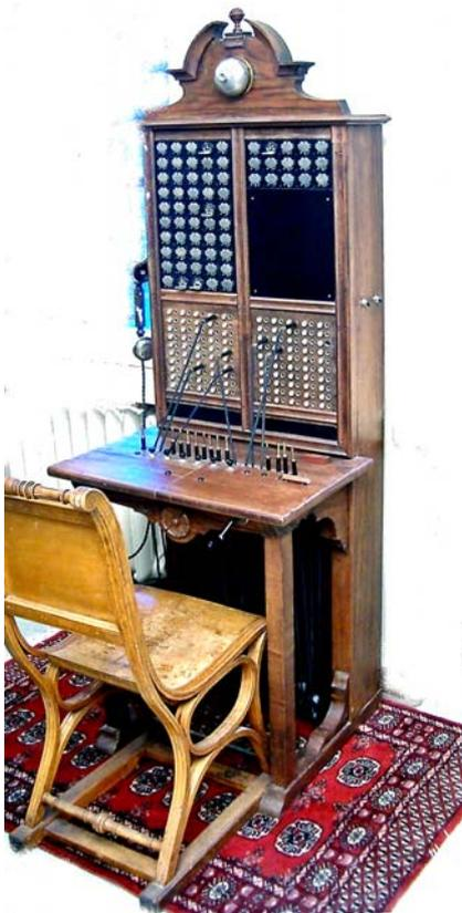
The equipment has been the switching board of some small telephone company near Helsinki. All the small companies in the Helsinki region united later to HPY. The chair in the picture is a HPY standard telephonist chair.
